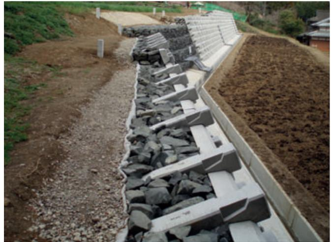
Fig. 5 and 6: Cross Beam Retaining Wall filled with crashed stones
