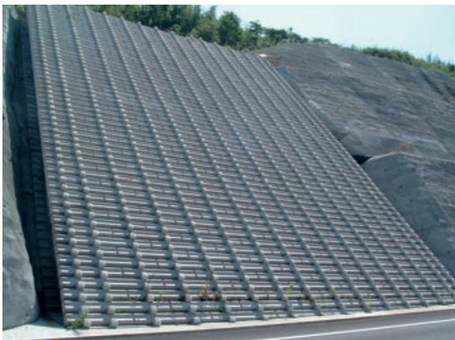
Fig. 2 and 3: Cross Beam Retaining Wall with precast concrete beams
