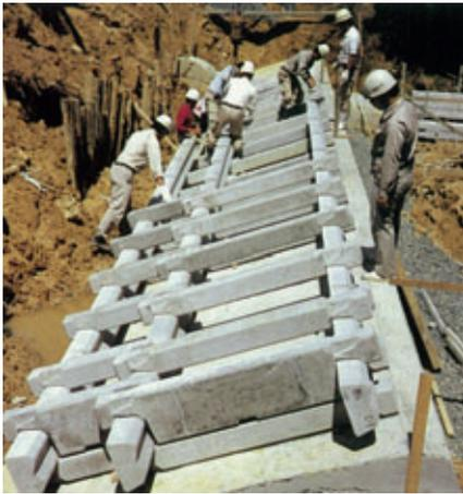
Fig. 7: Mounting of Double Cross Beam System
