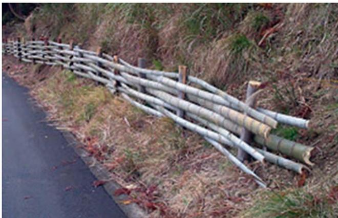
Fig. 1: A simple boundary fence “Shigara” which is made by bamboos and piles
